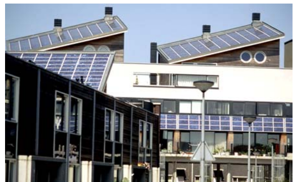
Fig. 6: PV-Roofs, Solar Settlement „Nieuw-Sloten“, Amsterdam, The Netherlands
