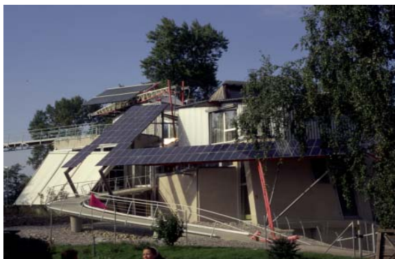
Fig. 3: Mansion, Breisach, Germany (Architect: Spiegelhalter)
