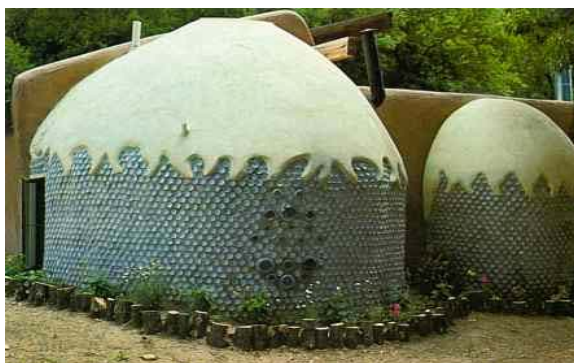
Fig. 5: Annex building out of tins, Taos, New Mexico
