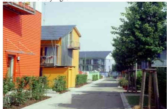
Fig. 12: PV-Roofs, Solarsettlement, Freiburg, Germany
