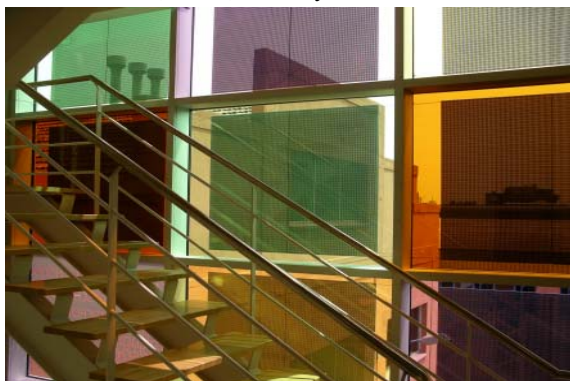
Fig. 10: Glass facade with semitransparent amorphous PV-Modules, Barcelona, Spain
