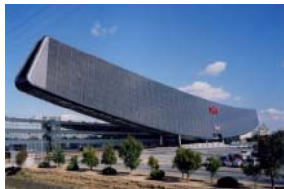
Fig. 8: Wall-cladding with crystalline PV-Modules, Solar Ark (Sanyo), Gifu, Japan
