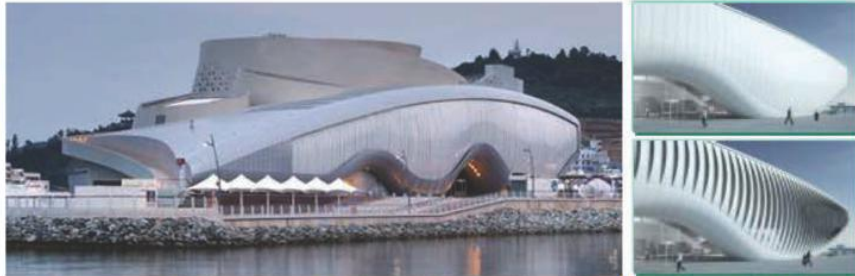
Biomimetic facade shading - Thematic-Pavillon Expo 2012 Yeosu, Süd-Korea
