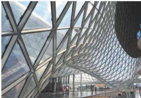
Ultra-lightweight support structure My Zeil Frankfurt: Support structure by Knippers Helbing Stuttgart
