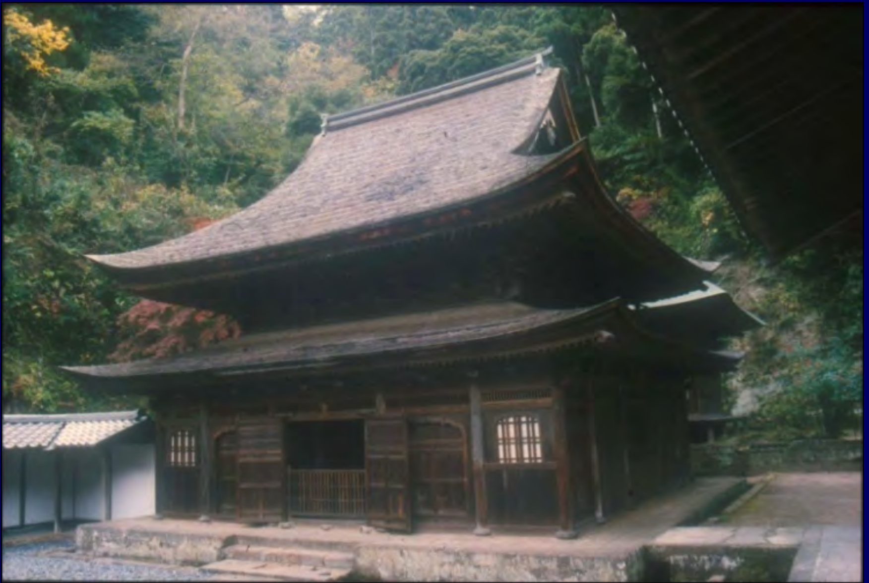
Engaku-ji Shariden restored after the earthquake (Photo by Prof. Sakamoto)
